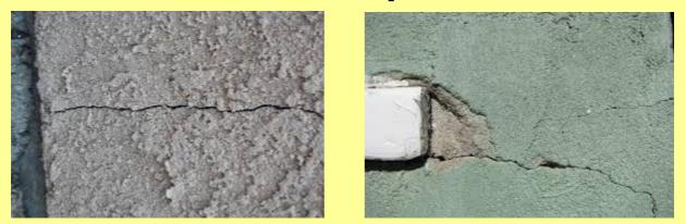
Cracked or missing stucco if not repaired will allow rain water in and more damage will occur.
